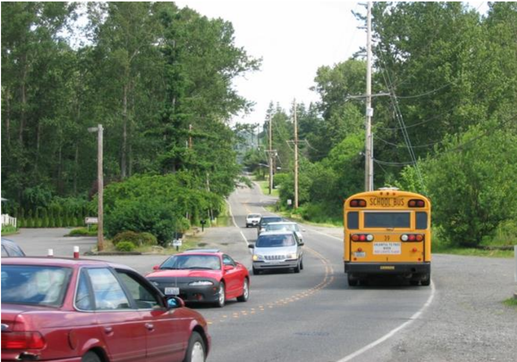
2013 Pre-Project: Deficient Bridge & Narrow Rural Roadway
